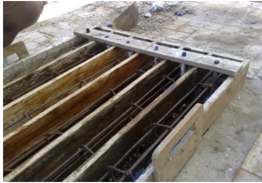
Figure (3): wooden pieces were fixed at formwork.
