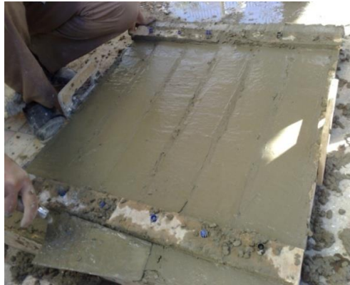
Figure (5): flattening the surface.
