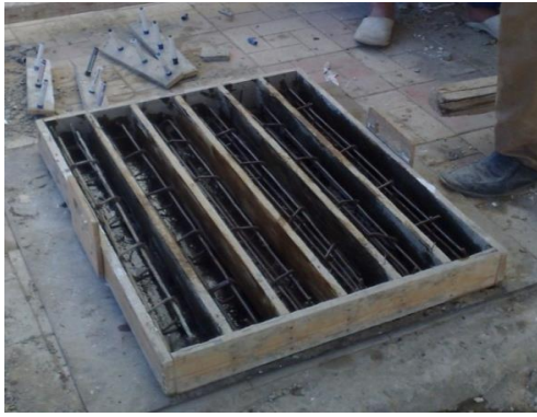
Figure (2): Formwork shape
